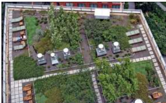
Azotea verde del Solaire, Nueva York, Photo Copyright © birdworks /Simon Bird and the Albanese Organization.)
